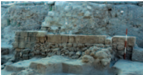
Figure 2.5: Wall 458 showing method of construction of exterior walls in Building 776 (view to east)
