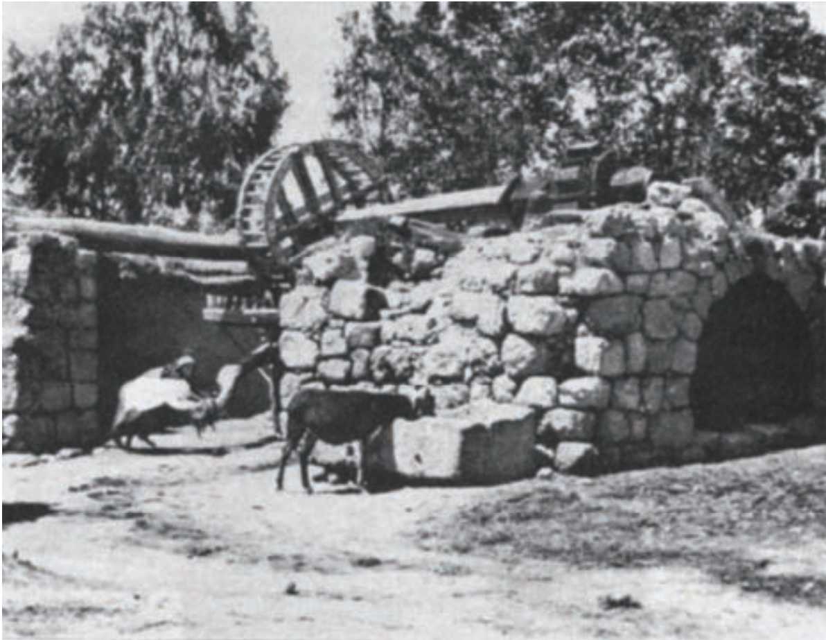
Figure 6.2: Coastal Palestinian well-wheel mechanism in use in the early twentieth century (Dalman 1932:photo 47)
