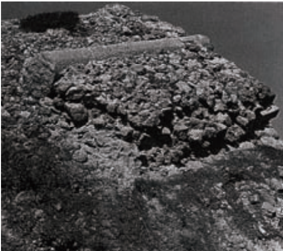
Figure 22.5: Detail of tower masonry
