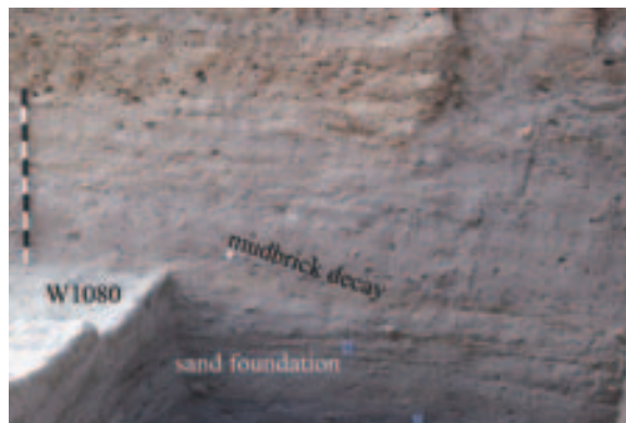
Figure 15.8: Section of Wall 1080; sand foundation is visible, along with mudbrick decay
