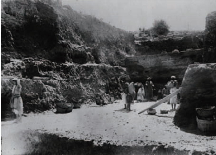
Figure 9.8: Step-trench excavated in the sea cliff by W. J. Phythian-Adams (view to east) Courtesy of the Palestine Exploration Fund
