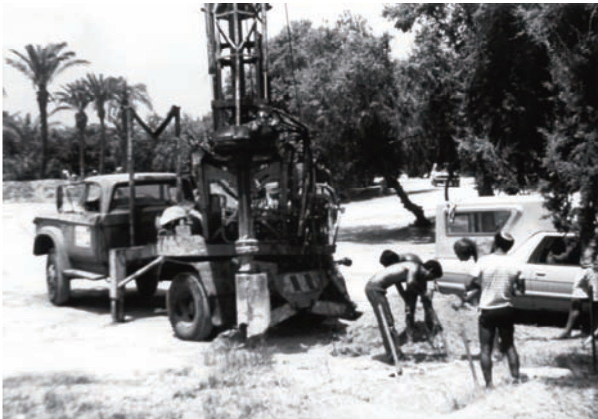
Figure 4.39: Equipment used for drilling core holes
